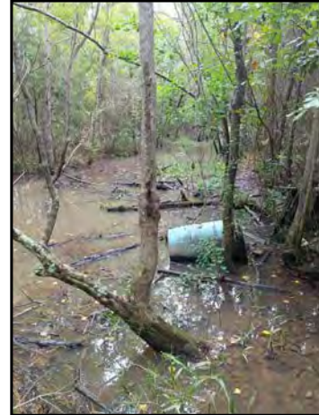
56 : PONDED WATER - NORTH CENTRAL DRAINAGE PATHWAY
