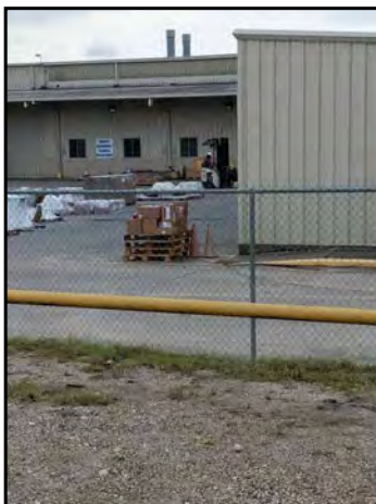
77 : TYP. BUILDINGS IN CANRIG COMPLEX - NORTH OF SITE
