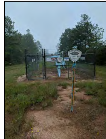
22 : LOOK. NORTH ALONG PIPELINE ON SITE
