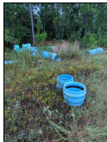
12 : LEFT OVER PIPE ON SITE
