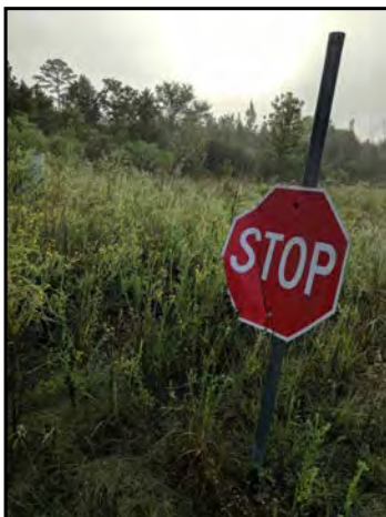
47 : ROADWAY/UTILITY CLEARING - WEST PART OF SITE
