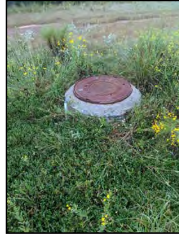
14 : MANHOLE - EAST PART OF SITE
