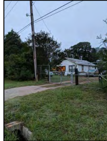
8 : HOUSE IN SE CORNER OF SITE
