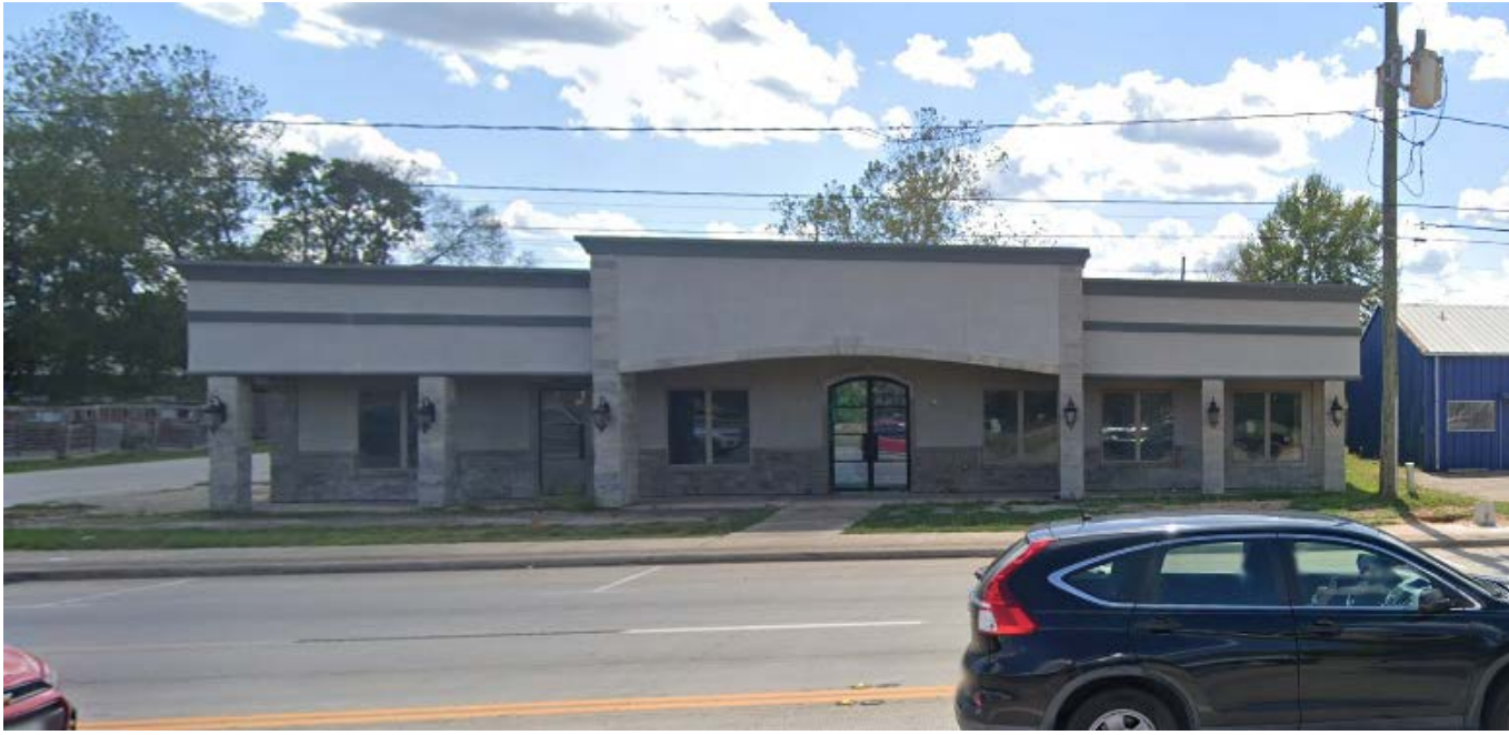
203 Magnolia Blvd. Legacy Mechanical Solutions (new)
