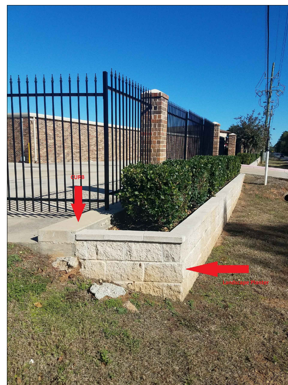
SECTION C - C LANDSCAPING PLAN AND SMU BLOCKS STEP-DOWN CONSTRUCT PHASE II FENCE ABOVE THE PROPOSED CURB AT 3 FEET FROM THE PROPERTY LINE AS A LANDSCAPE BUFFER - USING SPLIT FACED CMU BLOCK TO STEP-DOWN FROM TC ELEVATION TO THE LANDSCAPE PLANTER.
