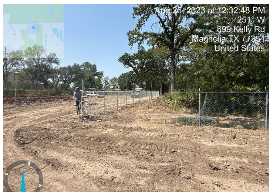
Site fencing improvements
