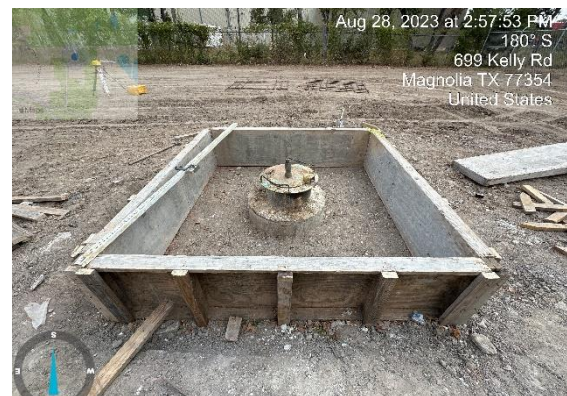
Water Well No. 8 and formwork for foundation
