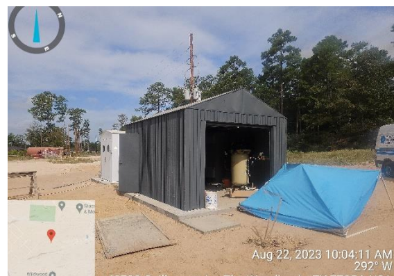
Temporary electrical and chemical sheds
