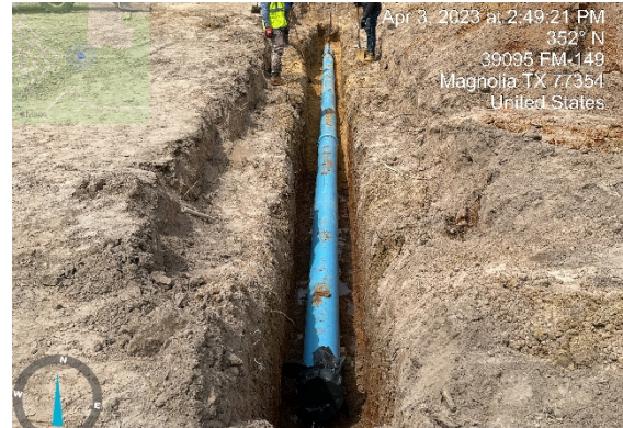
Water Line Under Future Mill Creek Road
