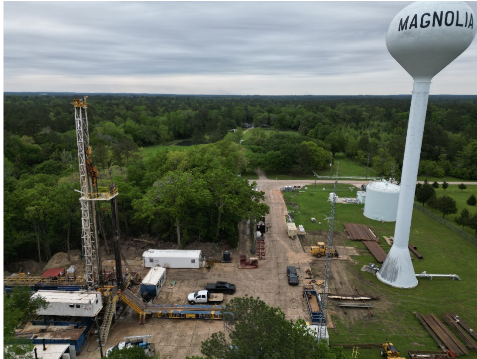
Drilling Rig and Water Plant Site
