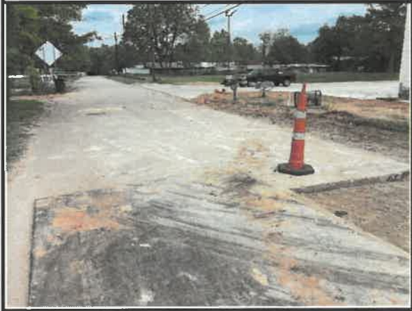
Restore site and replace asphalt along Roy St.
