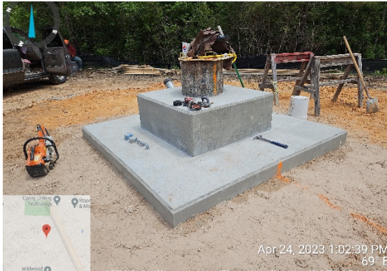
Water Well and Foundation
