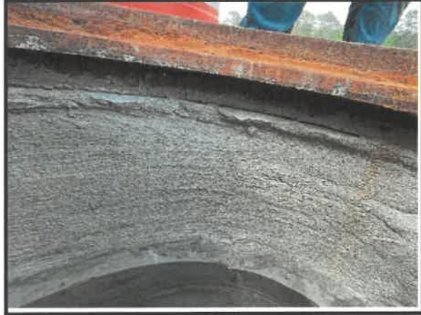
Fully seal ARV manhole ring.
