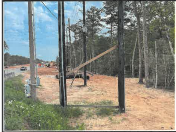
Verify CNP was informed of completed work.
