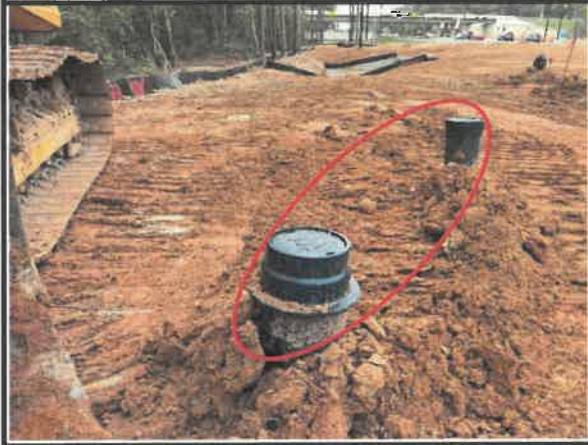
Ensure valve box is appropriately colored.
