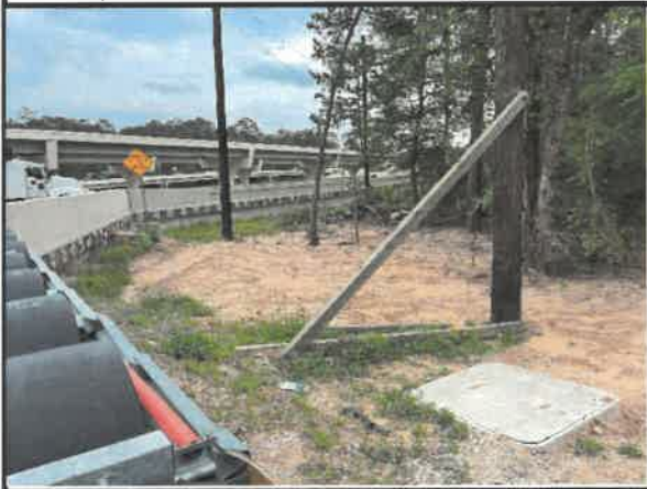
Verify CNP was informed of completed work.
