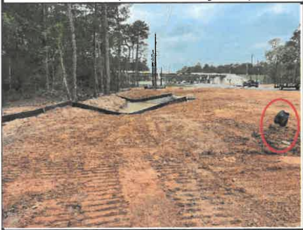
Remove and dispose of existing fire hydrant.
