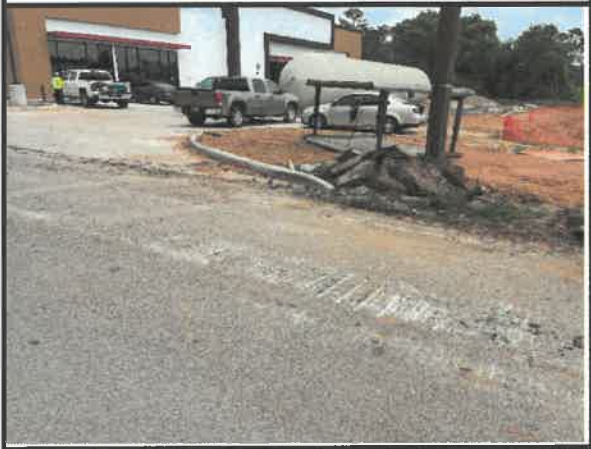
Restore site and replace asphalt along Roy St.
