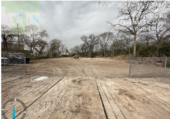
Cleared and grubbed well area
