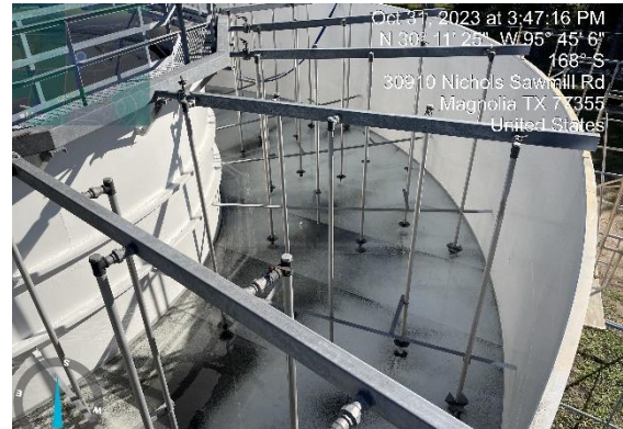
Coated tank walls
