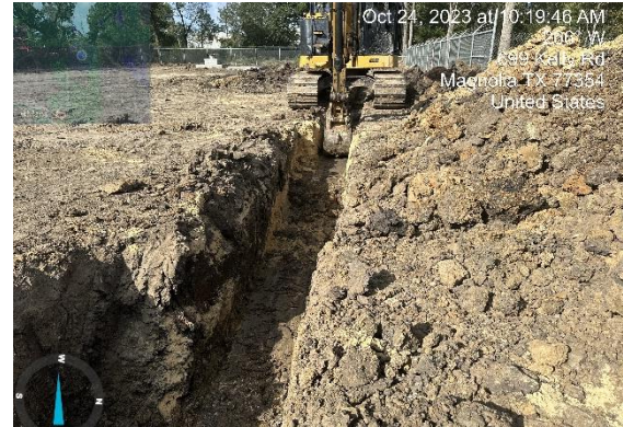
Trench for Well Discharge Piping
