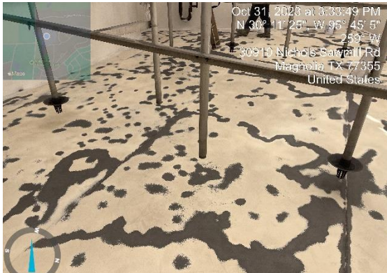
Aeration basin floor to be coated
