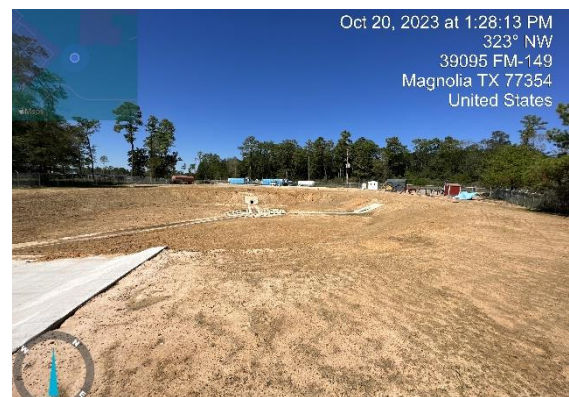
Detention pond and pilot channels
