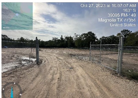
Detention pond and pilot channels
