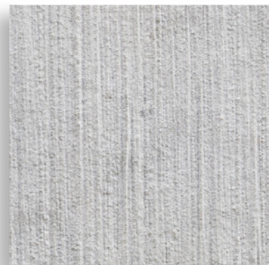
Light Broom Finished TILT-UP CONCRFETE WALL EXAMPLE
