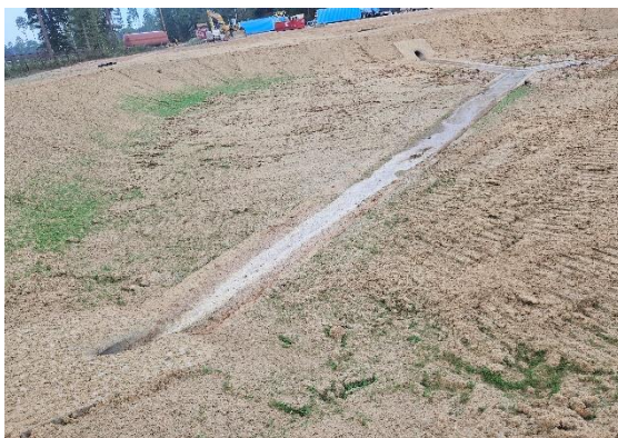
Detention pond and pilot channels
