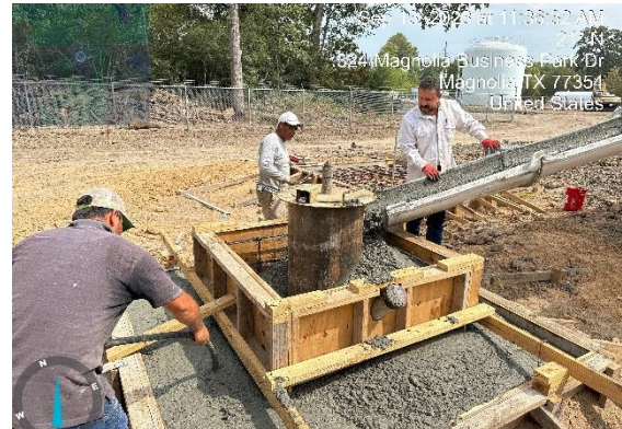
Water Well No. 8 and foundation
