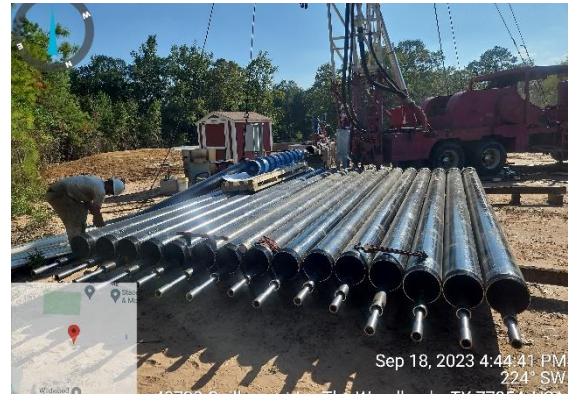
Column pipe assembly
