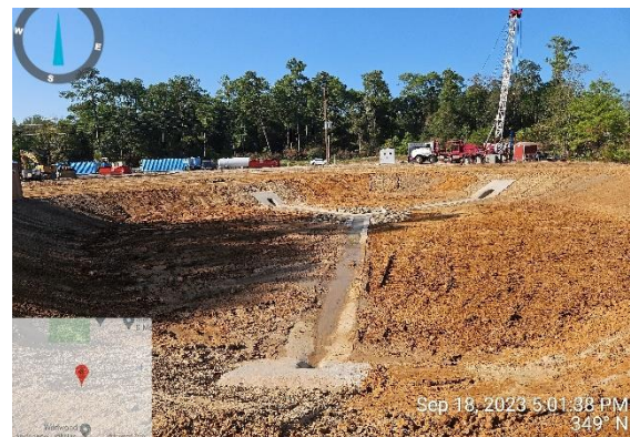
Detention pond and pilot channels
