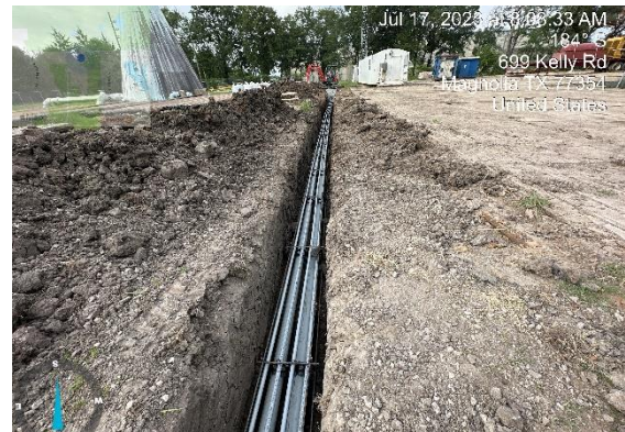
Electrical duct bank installation
