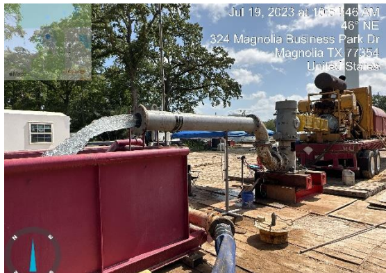
Water pumping for the step test
