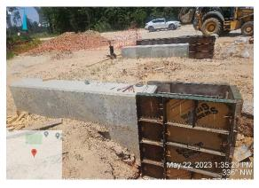
10,000-gallon HPT footing with formwork for cold joint extension for 20,000-gallon HPT
