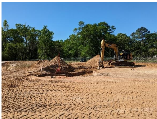
Preparation for GST foundation
