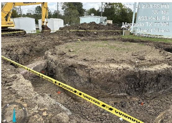
GST foundation subgrade
