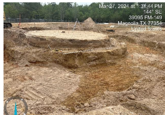
Preparation for GST foundation
