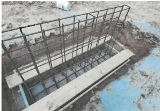
Rebar for HPT footing
