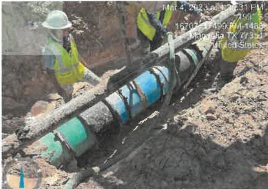
Repair of line
