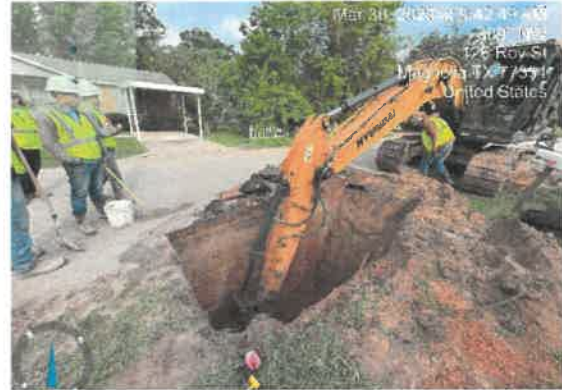
Connection near Roy Street lift station
