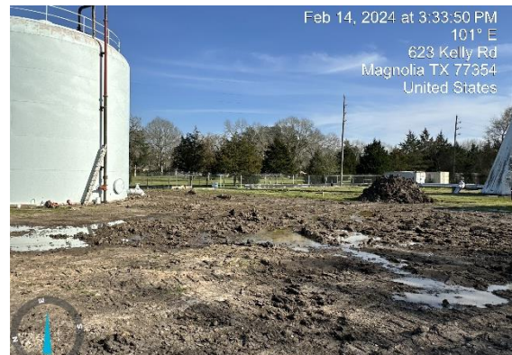
Water Well No. 8 fill line on existing GST
