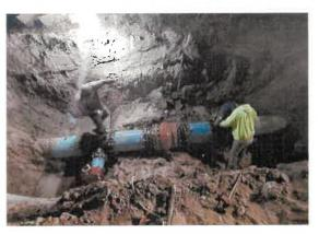
Check valve on 16-inch water line
