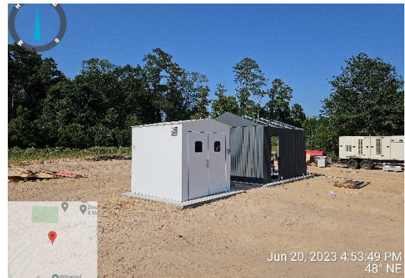
Chemical and electrical buildings
