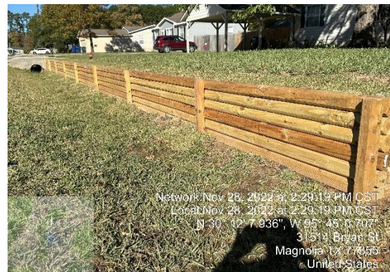
Relocated Timber Retaining Wall
